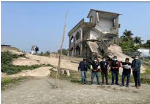
(c) Collapsed by riverbank erosion
