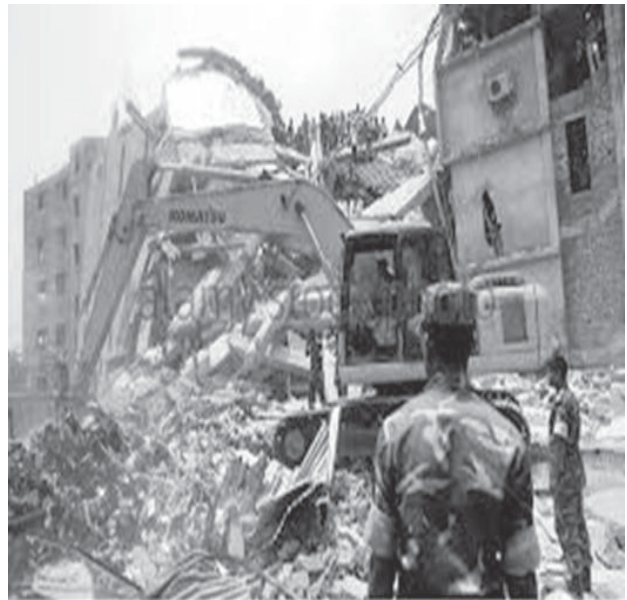
Fig. 2(b): Demolition by collapse
